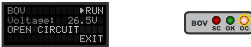
Figure 61 BOV Test - OPEN CIRCUIT
